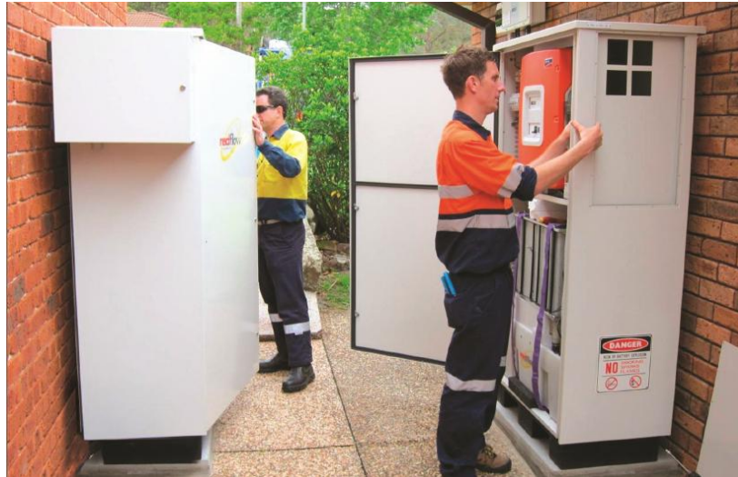
FIGURE 3: Two R510 ESS being installed in Newcastle
